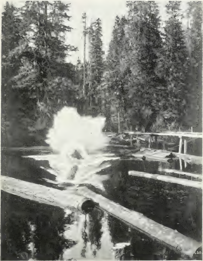
FIG. 65. TIMBER CHUTE : BRITISH COLUMBIA. [By courtesy of Canadian Government.]
